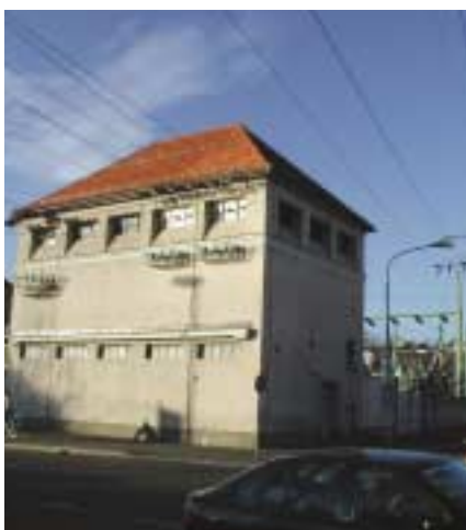
RTP 110 / 10 kV Melje
