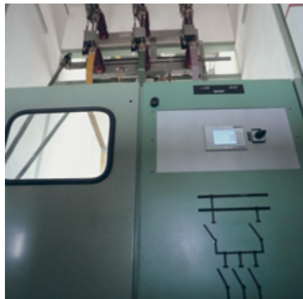
Shunt celice v RTP Ruše
