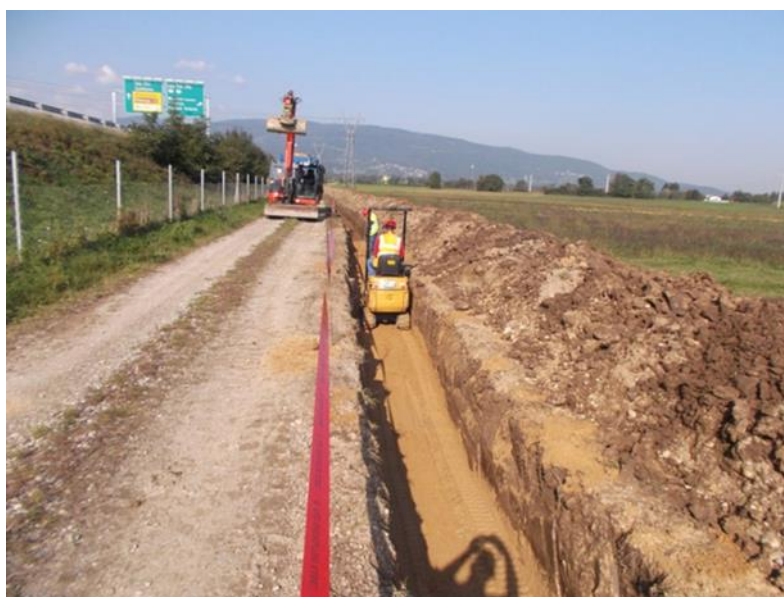
Figure 83: Works of Elektro Maribor d.d. for Magna Steyr
