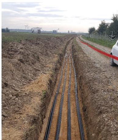
Figure 82: Cable line for Magna Hoče Nucleus
