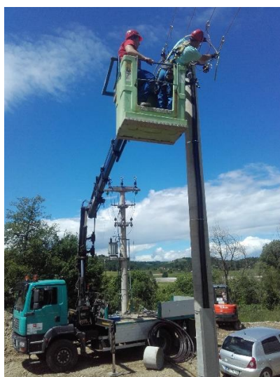
Figure 81: Works on Draženci Motorway - Gruškovje International Border Crossing
