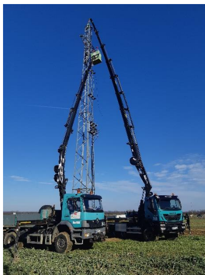
Figure 79: Dismantling of steel masts over the A5 motorway (Pomurje motorway)
