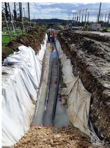
Figure 83: Laying cables in RTP Podlog
